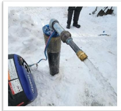
**Pump Installs:** We can install a pump through the top of the well while we are still drilling in the area. We offer a ½ hp, 115 volt, 3" submersible pump option (Grundfos 10SQ-series) that works great in 4" wells and with lower-wattage generators and solar. For deeper wells, a different pump may be needed. We drill a weephole in the drop pipe to help prevent freezing issues. Please see picture to see how the final well typically looks like with a pump install through the top.
