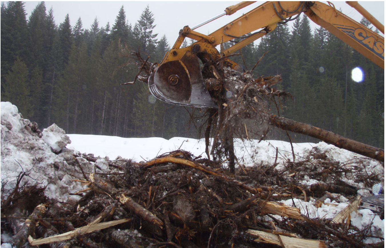
Figure 7 —An excavator is a good tool for building machine conservation burn piles. Dropping material from above keeps soil out the piles. USDA Forest Service photo by Jim Archuleta.
