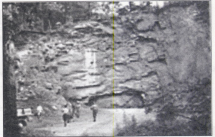
The quarrymen of Tohickon Quarry Company, circa 1939, head toward the quarry ledge. Stone boulders created by blasting down the face of the ledge with dynamite, had to be reduced to a size that would fit into the "crusher." This was done by using blasting caps on the large boulders and manually breaking up the smaller ones with a sledge hammer. Joe Long may be one of the men in this photo.
