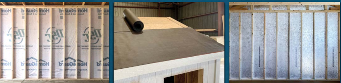
HOUSE WRAP VAPOR BARRIER | P1
