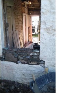
out, Iain built up the external wall in stone – like doing a jigsaw with pieces that don't really fit together at all! Then we lifted the sill back onto the top and bedded it in with mortar at the desired height for the new window. Lunchtime while things set a bit.
