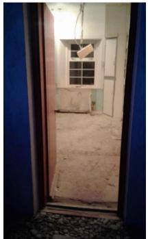
Took load of wood (old kitchen cupboard etc) to the tip in Stranraer first thing. Then continuing to take down the ceiling in the kitchen and clear the rubbish. Had managed to squeeze the plaster into the skip, but left with hundreds of laths to burn. Had a day long bonfire at the back of the field. Took all the old fibreglass insulation out of the loft and managed to load it all into the trailer with a sheet over everything to keep it in. Another load to the tip at the end of the day.
