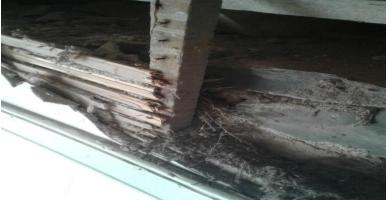
behind the dry-lining above the window and loads of wet rubbish in the coombes between the roof joists / rafters. Managed to clear much of this out, but so much that it was difficult to ensure there would be good ventilation for the roof-space. Maybe try hiring an industrial hoover?
