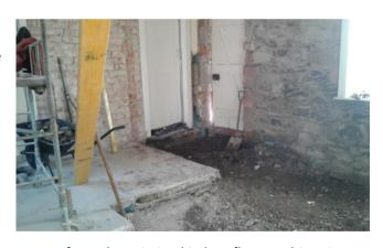
fireplace wall at the right level so we could level the concrete across from the existing kitchen floor to this using a long length of 4"x2" timber. Then, as we reach the front corner of the bedroom, the timber would be removed and the strip where it was is filled and floated to level off with the rest of the floor – and so on. Sounds good to me! We'll see if it works in practice tomorrow.
