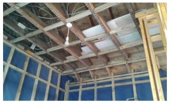
Early start again. Finished fixing the bedroom door frame and attaching the battens we need to be able to fix the plasterboard up to the frame on all sides. Then started putting in the noggins (Yorkshire) / dwangs (Scottish), between the ceiling joists to which the edges of the plasterboard will be screwed. Can't believe how much timber goes up in preparation for plaster boarding – I've cut miles of 2"x2" rough sawn timber over the last few days!
