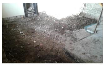
Only took about 20 minutes to take out the entire bedroom floor! Joists rested on a small 'foundation' at the front and back walls. No intermediate supporting foundations and joists basically laid on the earth. At each end, the earth was about half way up the joists and the joists were rotten. Nevertheless,
