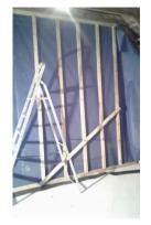
Started putting up new dry-lining on the bedroom walls. Got 2 walls done with me cutting timbers to length and Iain assembling sections which were then up-ended into place and fixed to the roof joists at the top and to the new concrete floor at the bottom. No contact with the stone wall at all! The frame has a damp-proof membrane fitted to the back of it
