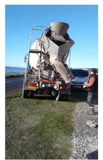
Measured up for concrete and calculated 1.1 m<sup>3</sup>. Decided we'd order 1.3m<sup>3</sup> to be on the safe side. Rang Luce Bay Plant to advise – "There might be a slight delay, the plant is frozen up this morning. We've been working on it since 07:00 but we haven't got the water flowing yet".
