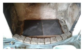
Laid two slate slabs as a base for the stove and then had lunch while the mortar set a bit.
