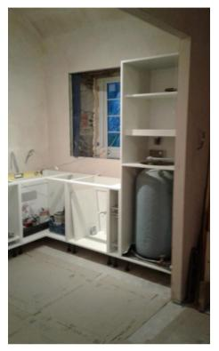
Doesn't sound much for a long day's work, but it isn't easy moving a tall unit about single handed! To take it in and out repeatedly during adjustment / trimming and fitting requires some ingenuity. Long timbers underneath the 'floor' of the unit, with the last one inserted while the unit is gently raised with a long lever, raise the unit by about half an inch to allow the unit to be slid in and out without breaking all the legs!
