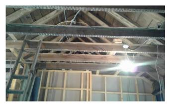
Did a bit of clearing up and covered all the tools etc. with old blankets prior to spraying the woodworm treatment. Mixed up 25lt of insecticide – it's not pleasant stuff so goggles, mask and gloves plus a boiler suit and straight into the shower afterwards.
