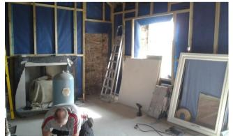
Got started just before 08:00 when Iain arrived. Straight on with dry-lining. Front wall and fireplace wall done by lunchtime. The fireplace is wrapped in black plastic sheeting to protect it while the plastering is done. It'll have a bit more sheeting added before the plasterers start, to protect all the front – although I've never seen plasterers who make as little mess as these guys!
