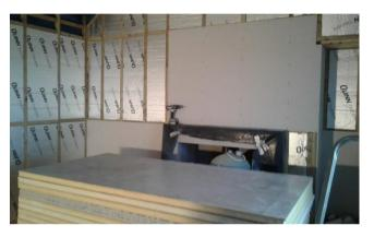
angle bead (for outside corners prior to plastering), and enough 'space blanket' to insulate 22 sq m of stud walls around the kitchen.
