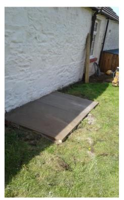
Plasterers arrived 08:30. Soon as they were started, got on with mixing concrete for the base of the shed. Used up the left over sand/gravel mix and then just used sand and gravel off the beach! Had to nip into Glenluce for more cement.
