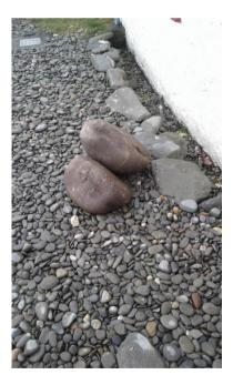
Riddled some of the sub-floor to produce some fine 'soil' to use as a soft layer immediately under the damp proof membrane. Stops it being punctured during the floor-laying process. Note the large stones!
