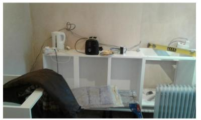
You can see the two clamps holding the cupboards temporarily in place while I mark the positions of all the pipework. The cupboards then come out while everything is connected up in the right place. If I get any leaks, it'll be a major job taking everything out again to fix them!
