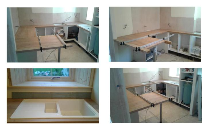
All ready for me to fit the sink and hob. Fortunately, I have clamps, so left the clamps on a couple of timbers holding the edging strip which has to be glued to the back of the worktop that forms the breakfast bar. Leave those until the morning when the glue should have set nicely.
