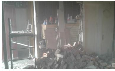
Started taking down the living room / kitchen wall. The poor quality photo is actually the dust in the air! The door on the right is the old door into the kitchen. The scaffolding is in the hallway with the doorframe of the living room door just visible 'framing' the scaffolding.
