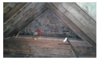
Took nearly 3 hours to spray the whole roof, sarking (the boarding under the tiles), ceiling joists and rafters. Not a pleasant job! Hopefully, we'll have a few less woodworm around in the hatching season in the Autumn. Interestingly, they'd gone for the rafters and joists mainly. I'd have expected to find most in the sarking but actually very little there. Maybe too cold just under the tiles?
