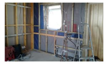
Rest of kitchen stud walls done after tea with the openplan 'flying wall' made up as a reinforced frame and then lifted into place before being fixed to the ceiling joists. Just a few odd bits and pieces to do tomorrow before we
