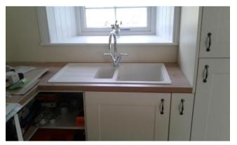
Fitted taps and waste to the new ceramic sink. It tells you to knock out the part pre-cut hole for the tap with a hammer and chisel. Bit reluctant to do that, but that's what I had to do in the end and it worked fine. Fitted the wastes and overflow. Connected up the hot and cold and tested it. One small leak on the u-bend but sealed that and everything seems fine.
