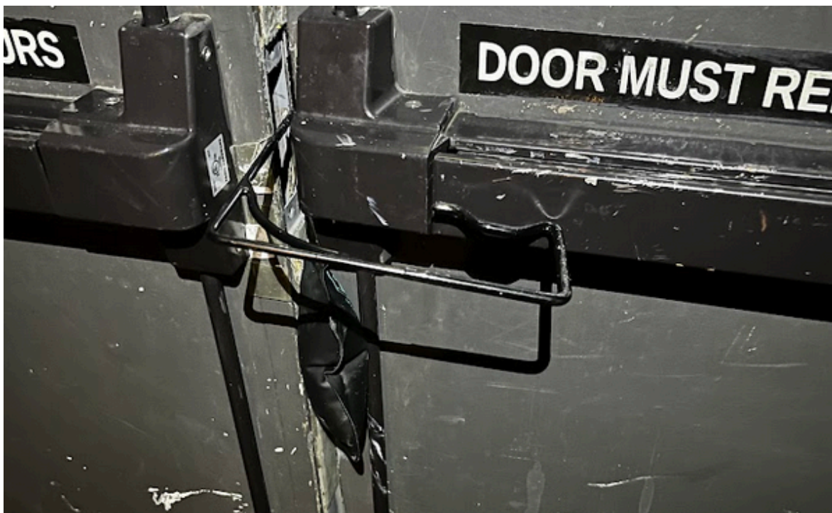
Figure 6b: Inside angle of the Double Door Tool hitting the crash bar
