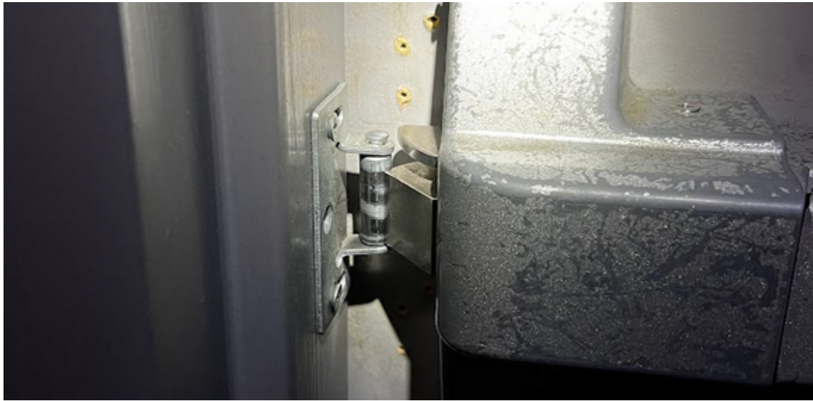
Figure 30: Front Vestibule door's latch barely sitting on locking bar
