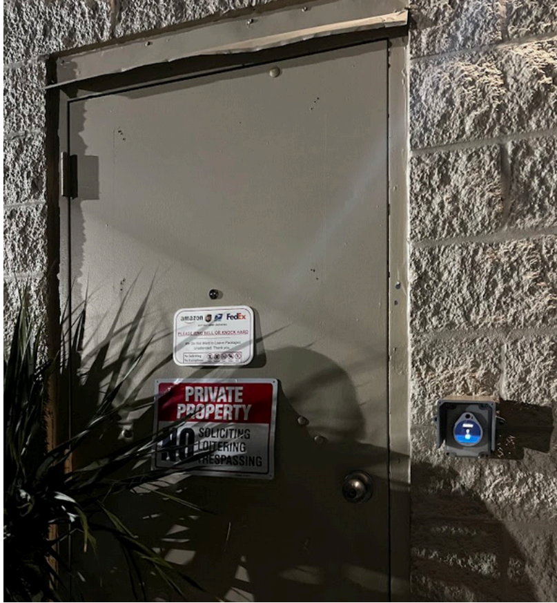
Figure 10: Employee Door, showing access control panel and exposed insecure hinges
