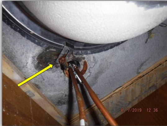
WET BAR SINK LEAK
