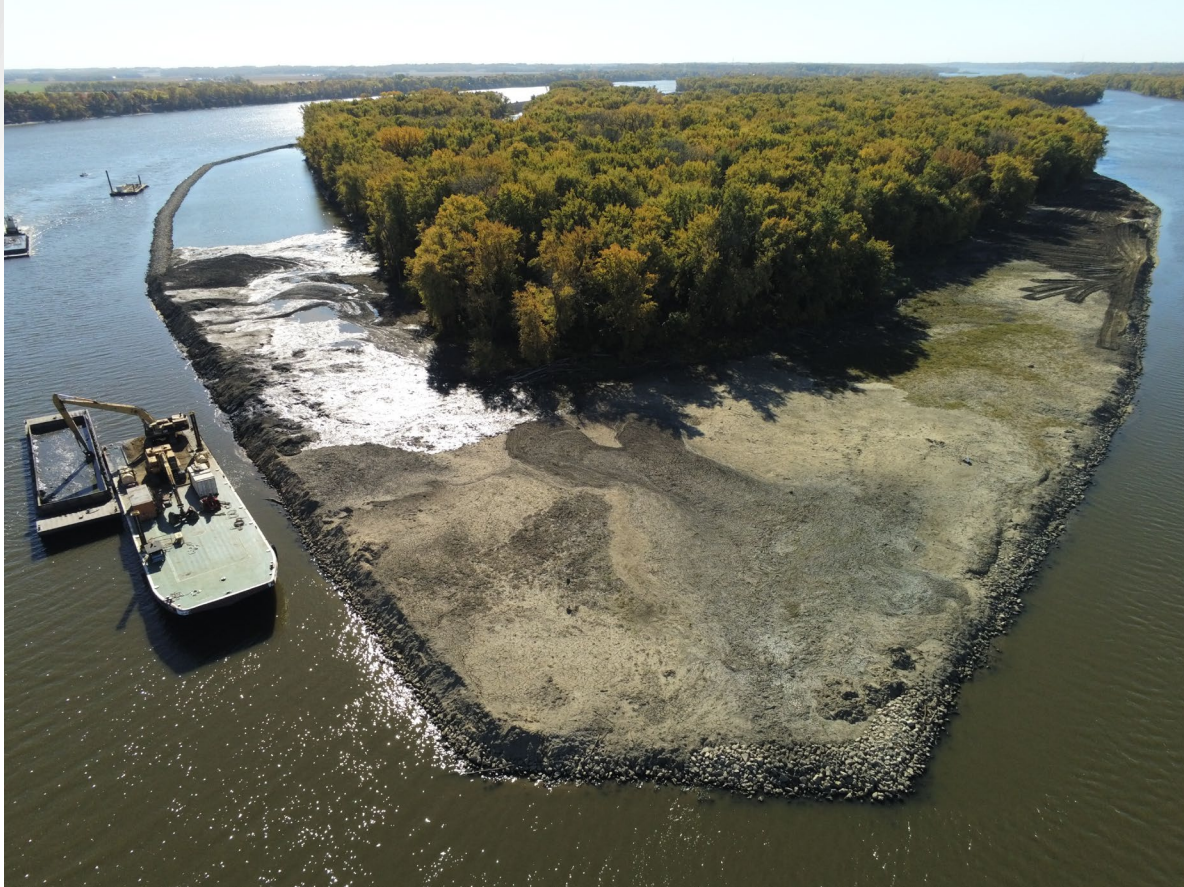
Head of Island Placement Progress 10/24/2024
