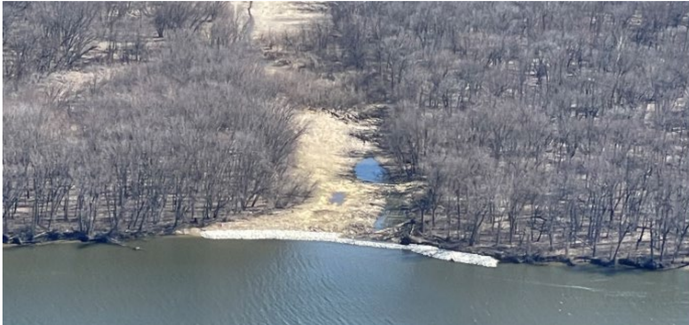
Grade Control Structure
