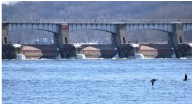
Lock and Dam 14
