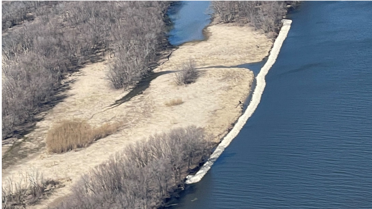
Northeast Bank Rock Placement
