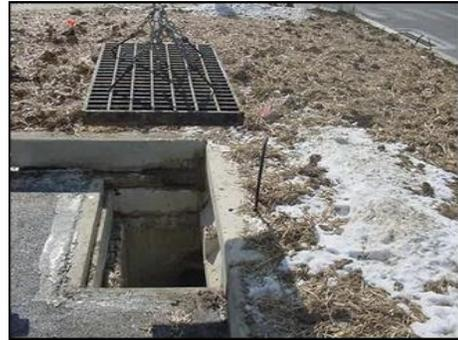
Attach Suspension Hardware to Rib of Storm Drain Grate
