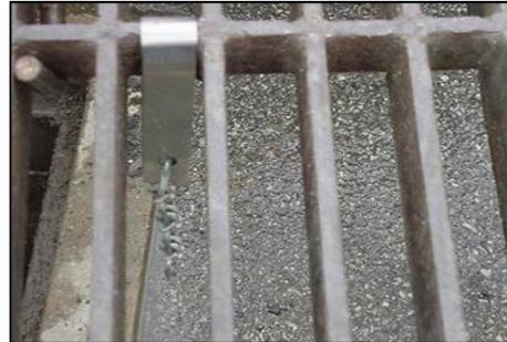
Attach Suspension Hardware to the Inceptor and Position Deflector Plate on Lip Where the Storm Drain Grate Rests
