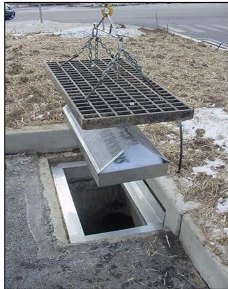
Carefully Lower the Grate with Inceptor Suspended into the Catch Basin
