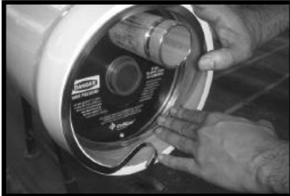
Installing retaining ring
