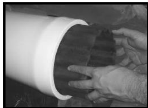
Installing thrust ring
