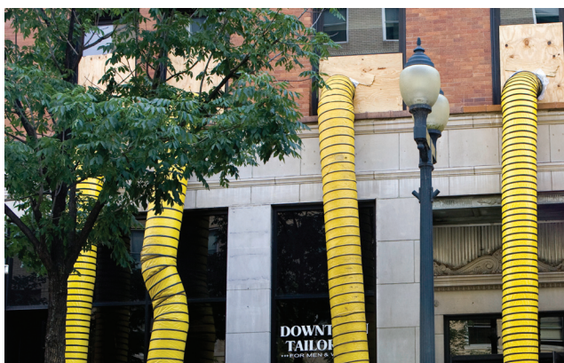
Cedar Rapids, IA, June 29, 2008—These large yellow tubes are used for drying the inside of flood or water damaged buildings so that repairs and reconstruction can begin. Courtesy: Susie Shapira/FEMA
