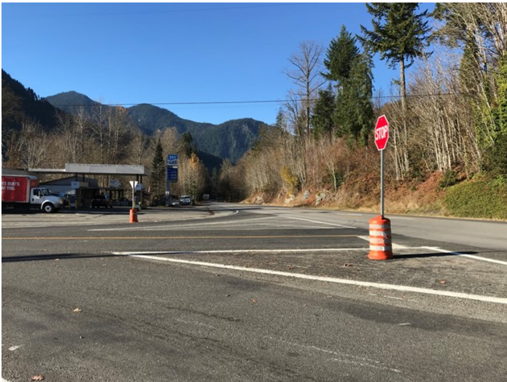
US 2 Existing Conditions at 5th Street, looking West
