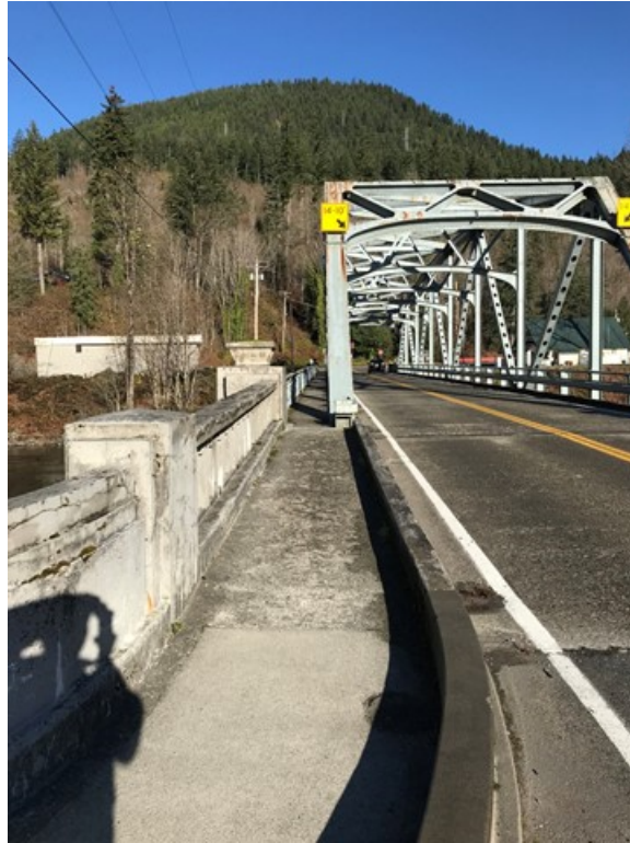
Pedestrian Sidewalk on 5th Street Bridge to US 2
