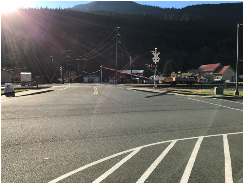
5th Street crossing of BSNF Railroad
