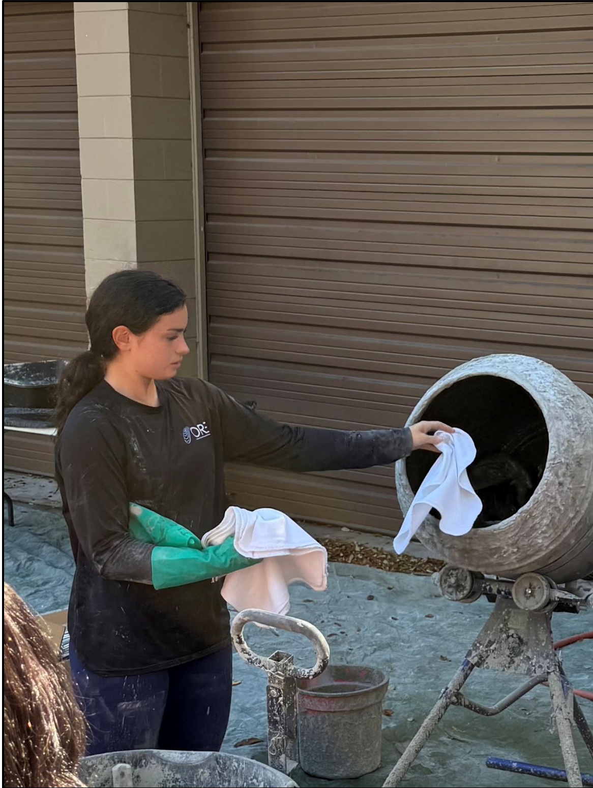
Figure 2 – Placing rags into the cement mixer one at a time
