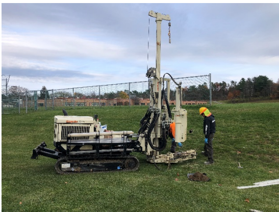
Drill rig collecting soil and groundwater samples at Algonquin Middle School
