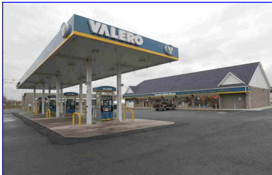
At a brownfield site in Lackawanna, NY, 6,000 tons of contaminated soil and several underground storage tanks were removed. The site was then redeveloped into a full service gas station.
