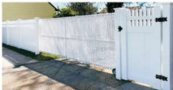
VINYL FENCE W/ CHAIN LINK SLIDING GATE
