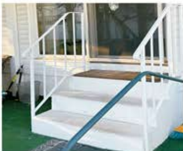
WHITE IRON RAILINGS
