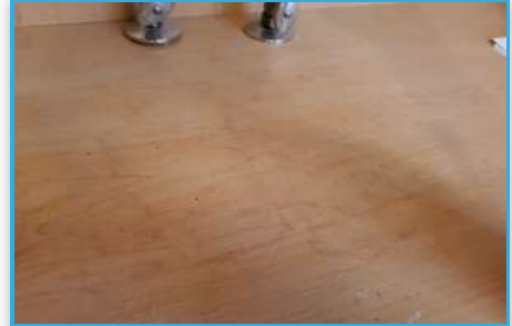
Location: MASTER BATHROOM
