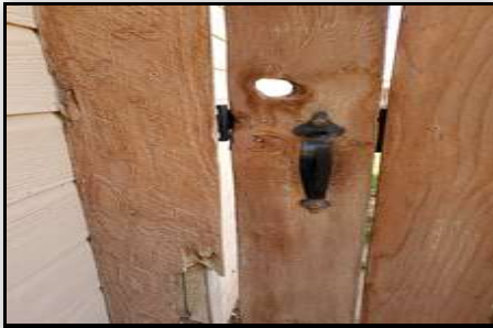
Location: NORTH EXTERIOR
