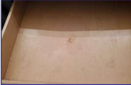
Location: MASTER BATHROOM
