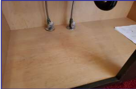
Location: MASTER BATHROOM
