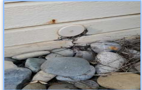
Location: WEST EXTERIOR
