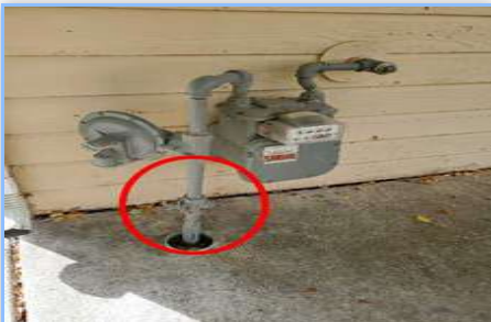
Location: NORTH SIDE OF GARAGE
