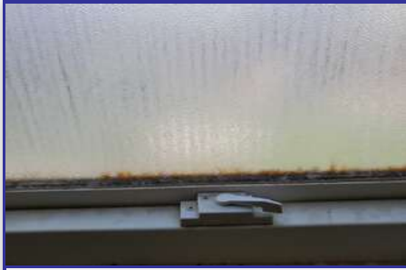
Location: MASTER BATHROOM
