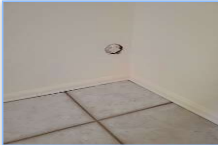
Location: LAUNDRY ROOM
