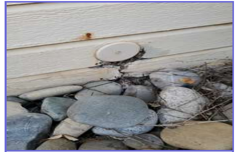
Location: WEST EXTERIOR
