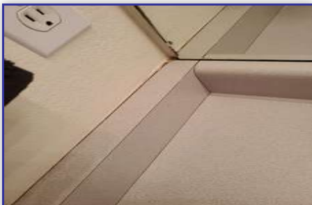
Location: MASTER BATHROOM
