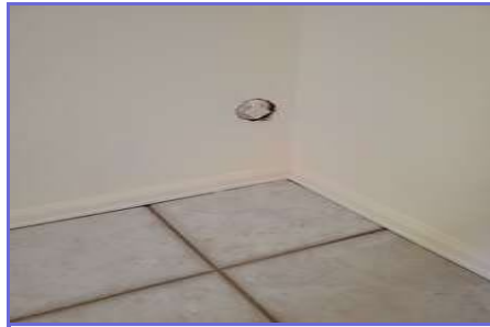
Location: LAUNDRY ROOM
