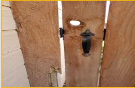
Location: NORTH EXTERIOR
