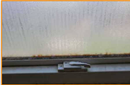
Location: MASTER BATHROOM
