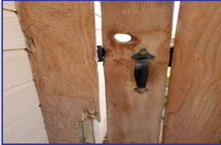
Location: NORTH EXTERIOR
