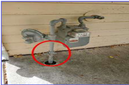
Location: NORTH SIDE OF GARAGE
