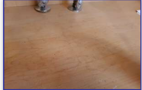
Location: MASTER BATHROOM
