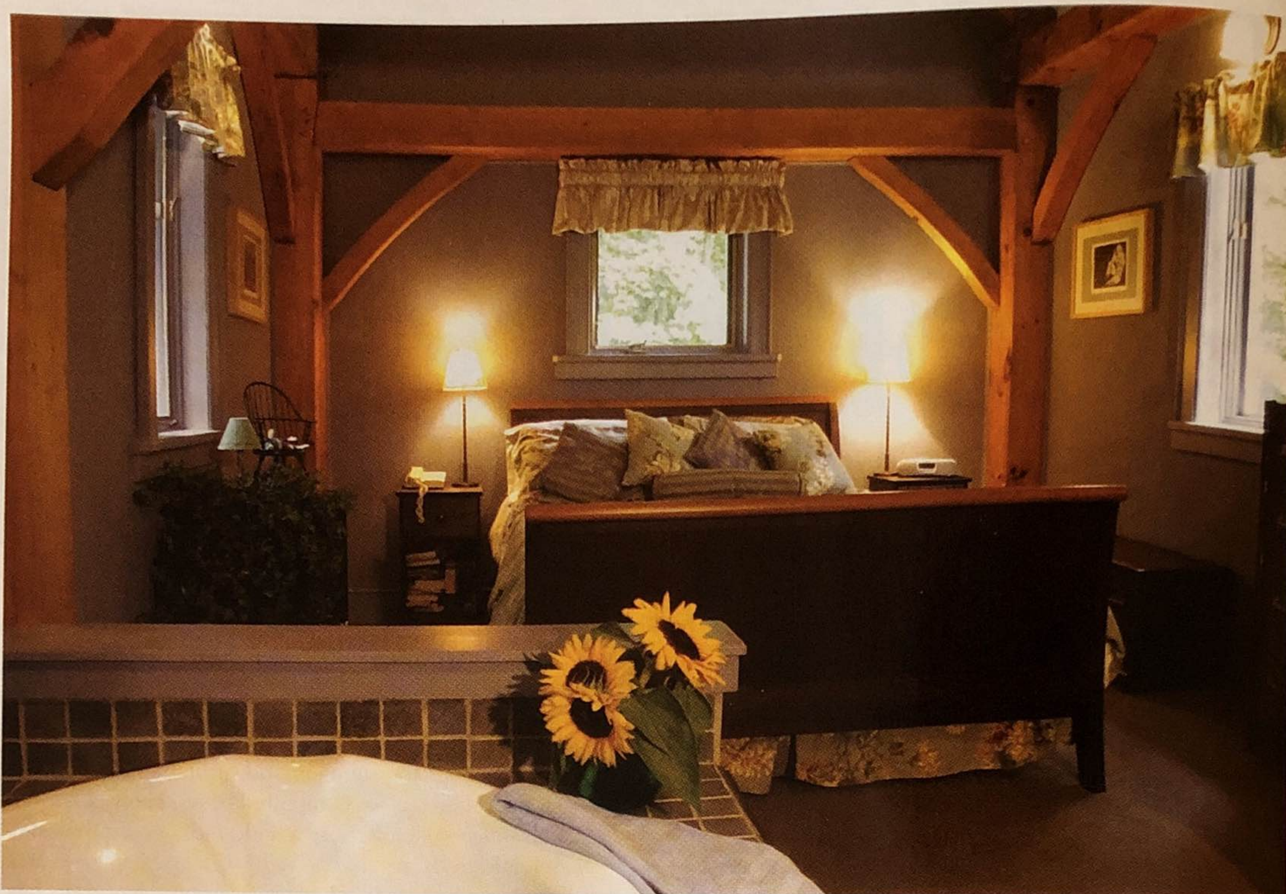
Two 10X20-foot timber frames were added to the original log home. One was incorporated into the kitchen area and the second (our bedroom) included windows on three sides and a door (see below) leading to a rear deck.
