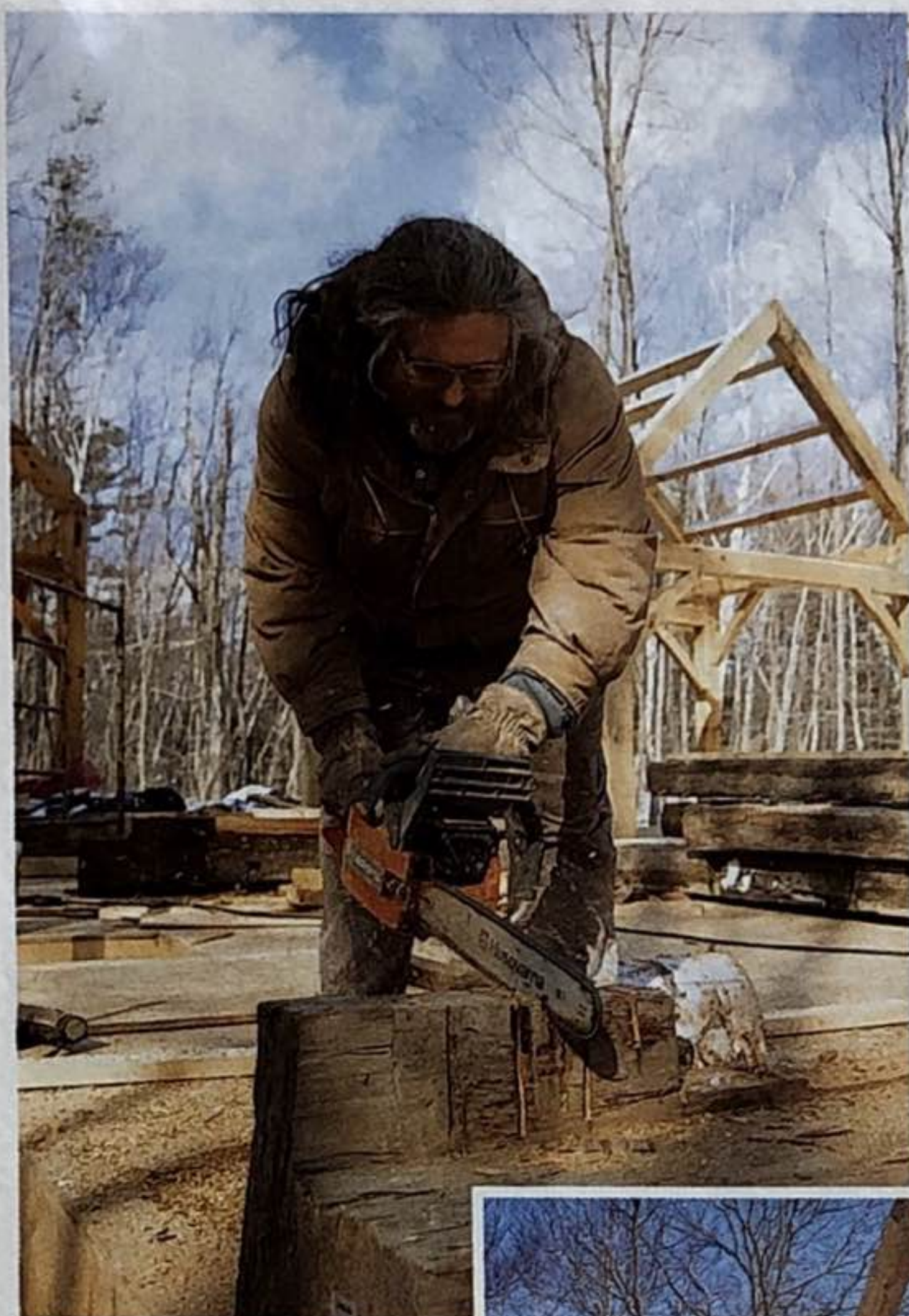
(Top) Bob Slater prepares the front base log. The log had to be levelled to sit evenly on a new foundation.
