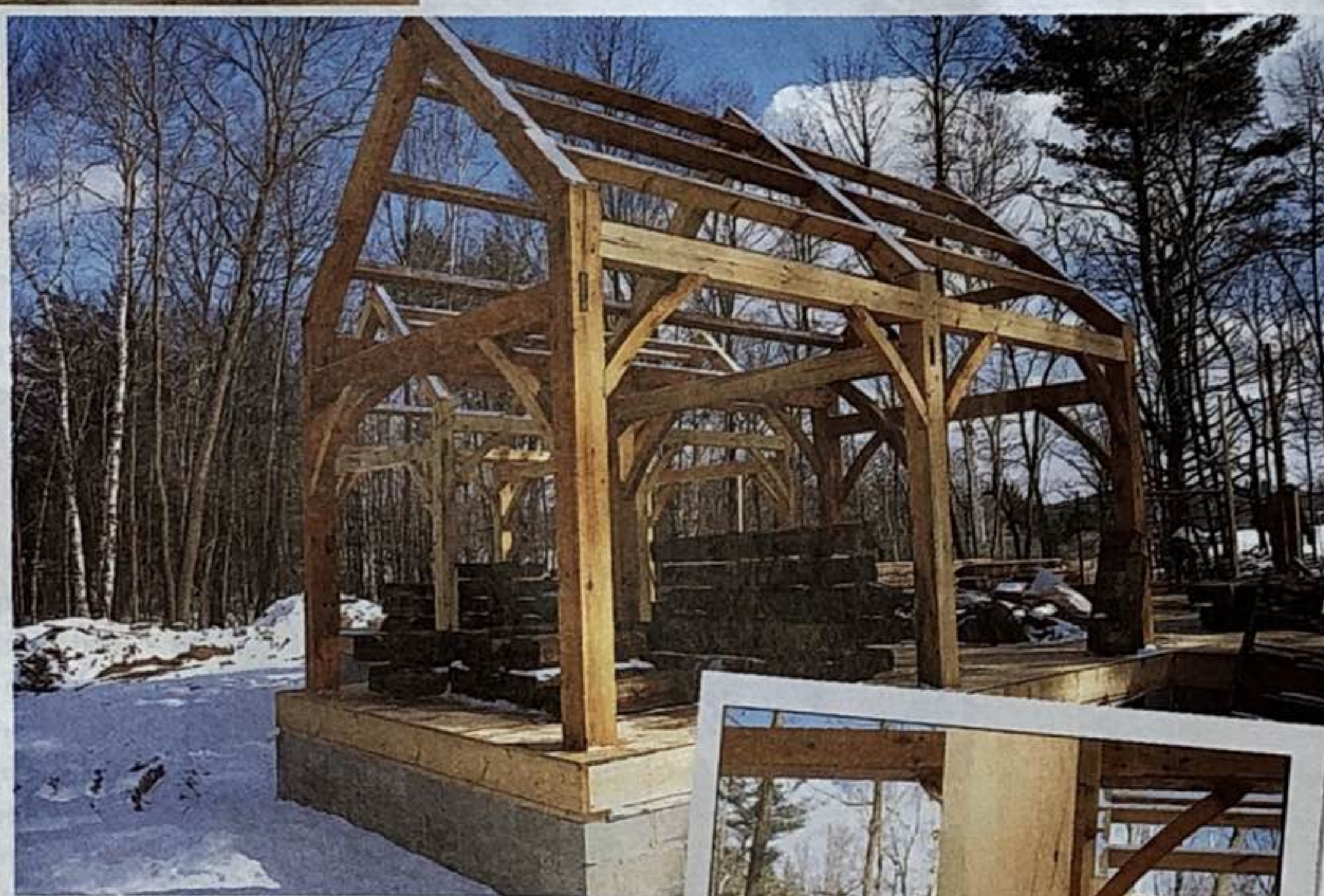
(Top) Bob Slater prepares the front base log. The log had to be levelled to sit evenly on a new foundation.
