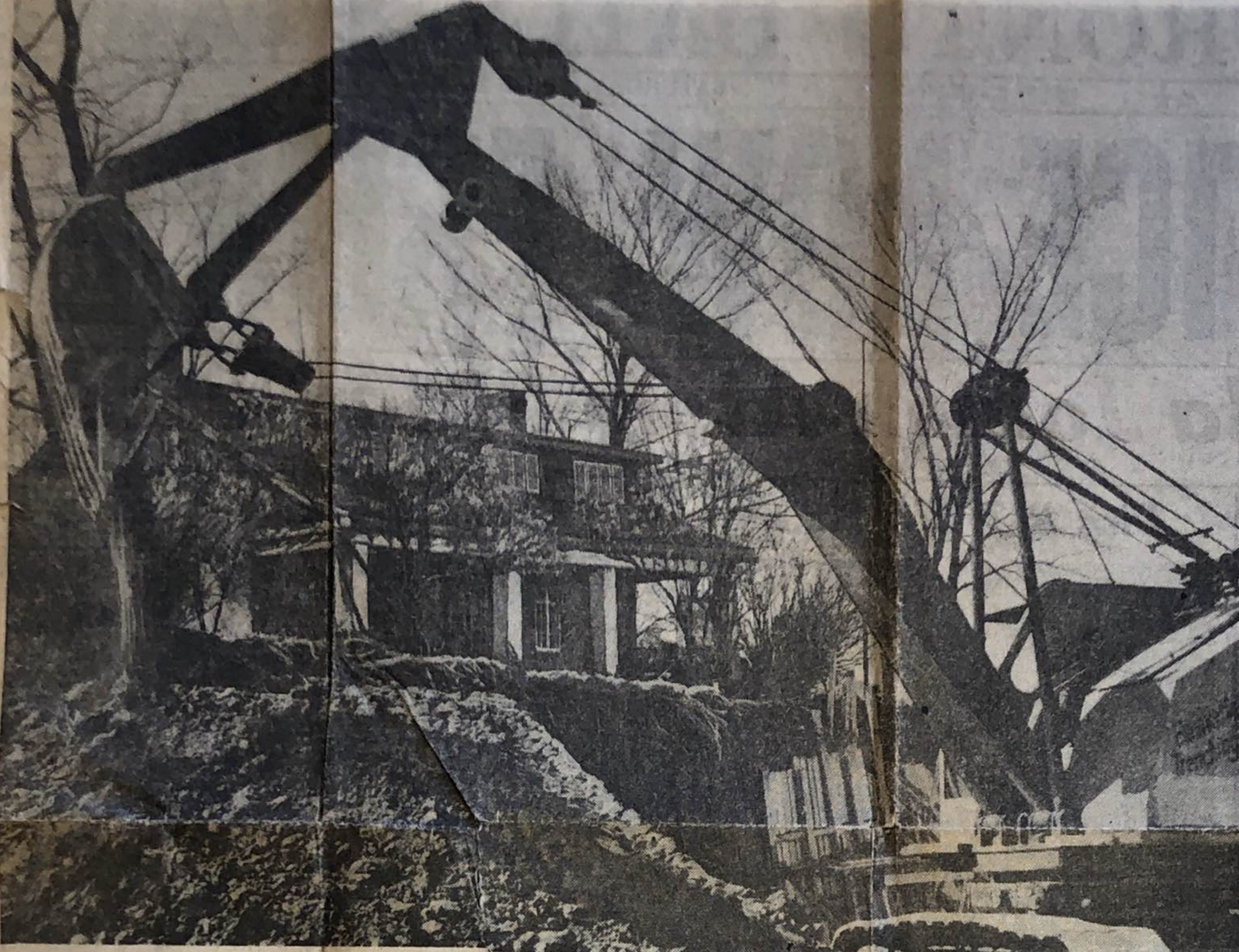
POWER SHOVEL at work excavating for a 44-suite apartment building at Bathurst St. and Ridelle Ave., is digging huge hole in ground and is source of worry to Mrs. Dora Mayor Moore, owner of historic 140-year-old house adjacent to excavation. She claims three of four feet of weeping tile has been cut into and the efficiency of her septic tank has been impaired
