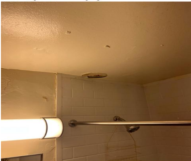
Betances - Construction Complete
