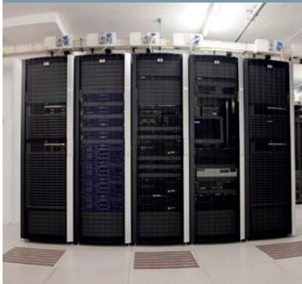
Safe Host data center in Geneva
