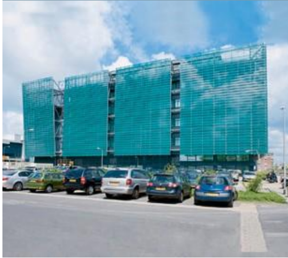
KPN data center in the Netherlands
