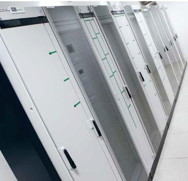
Totally Integrated Power from Siemens
