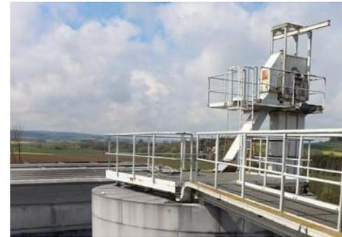
The Sitrans LR560 radar-level transmitter can reliably and continuously determine the filling level of the cullet silo over the entire silo height.
