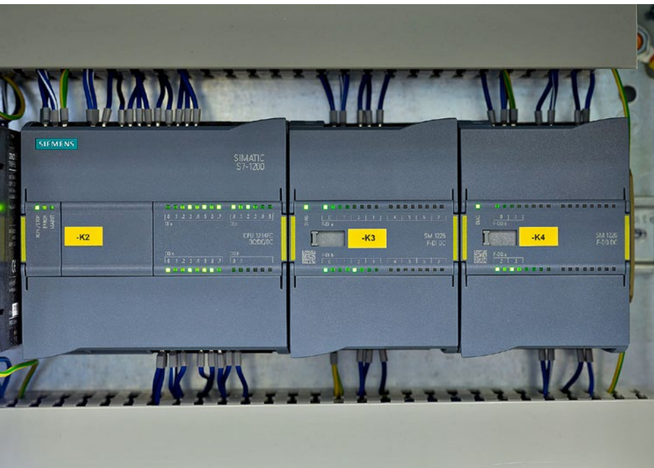
Thanks to the Simatic S7-1200 fail-safe controller, Möller does not need to wire an additional safety system
