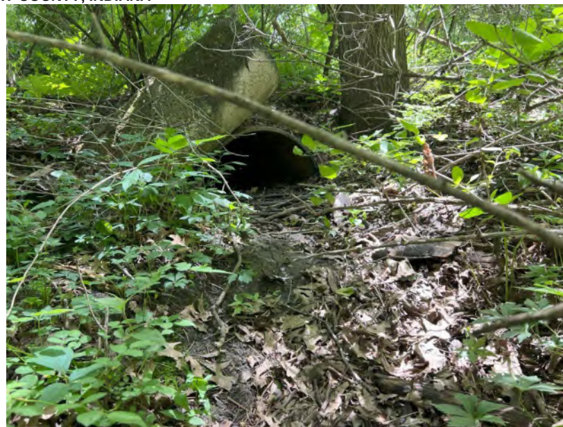
35. View south of culvert under the railroad. 6/6/2024.
