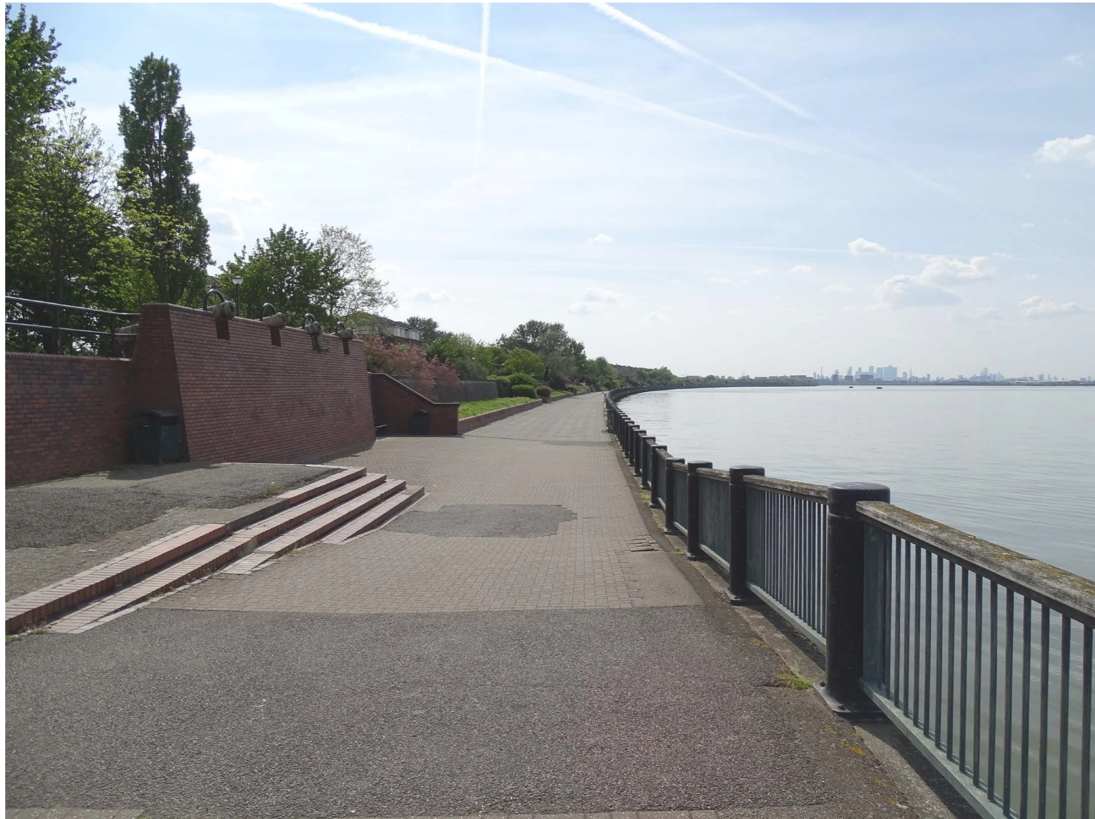
Crossness Explosives Piers along the Thames Path once home to a dangerous export is now a peaceful place for residents of Thamesmead to fish, cycle, walk and run. This creates a gathering point for a recreation area for residents.
