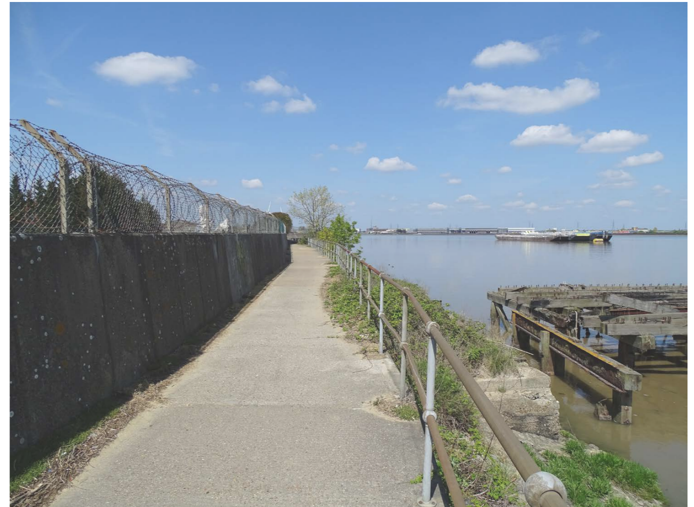
Concrete wall protecting the public from the concrete processing plant / Abandon Piers - Belvedere Industrial Estate.
