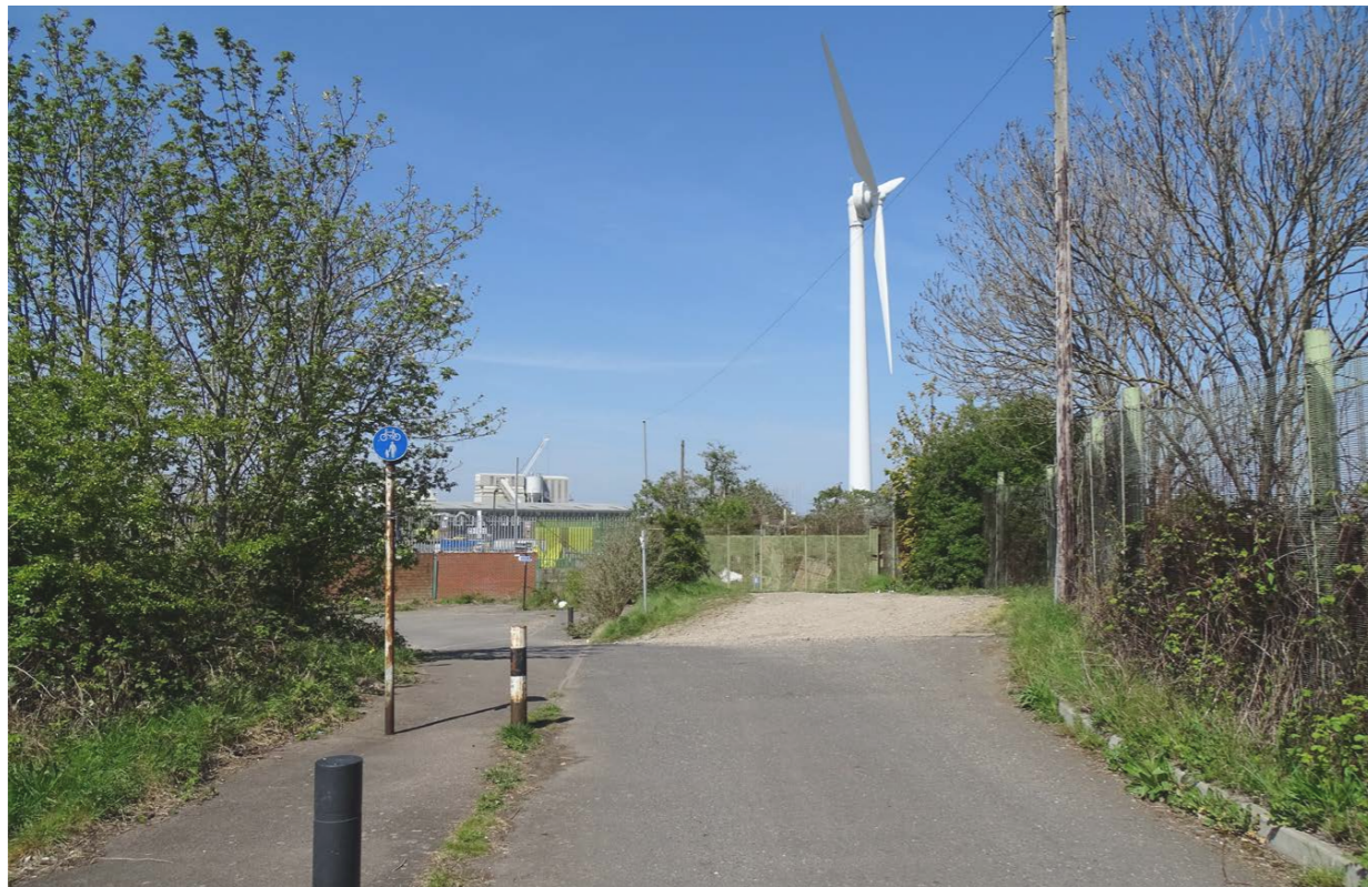
Anchor Bay Wharf, Erith.
