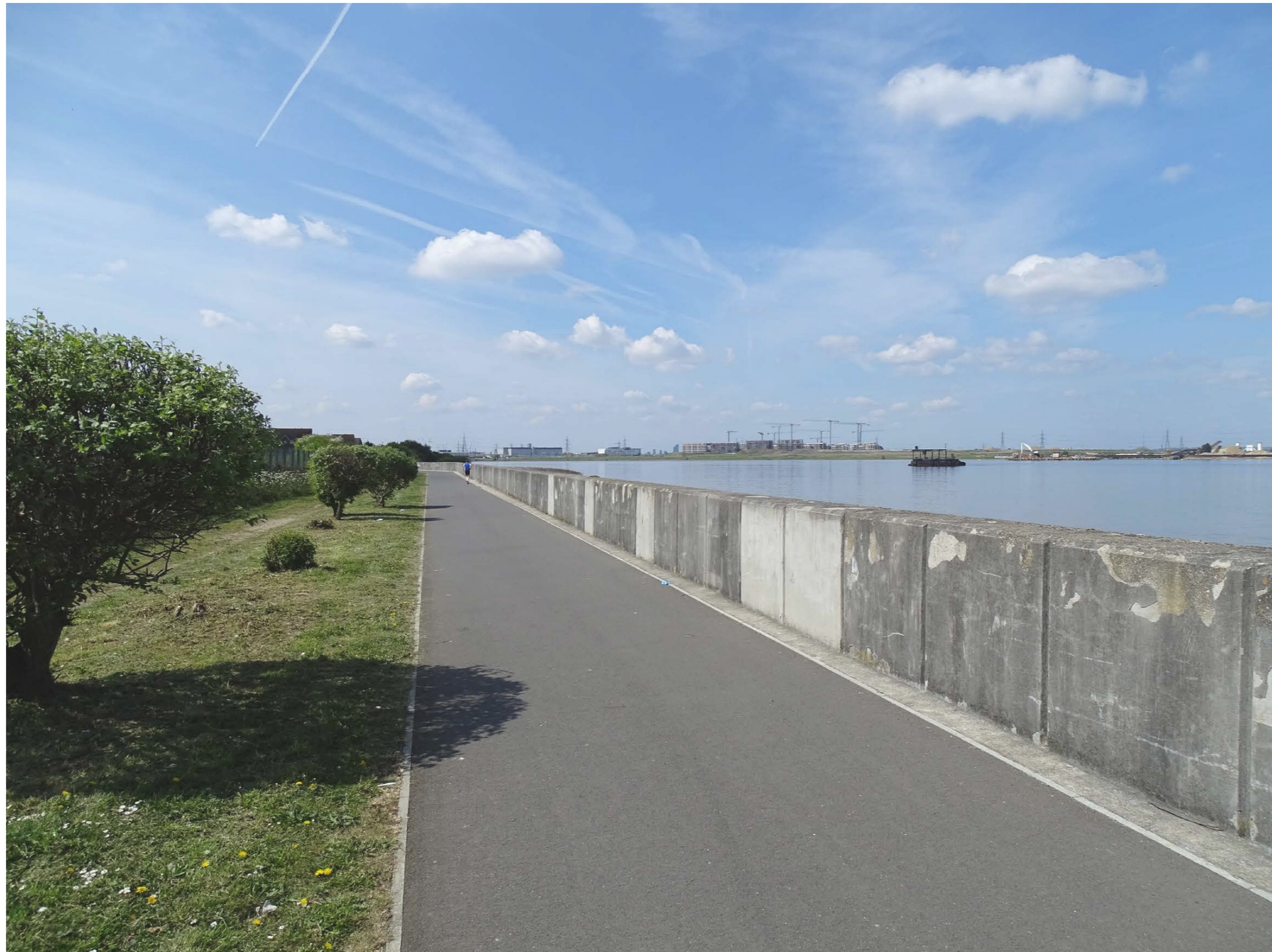
Thames Path alongside Ridgeway Park and Golf Centre with concrete flood barrier wall.
