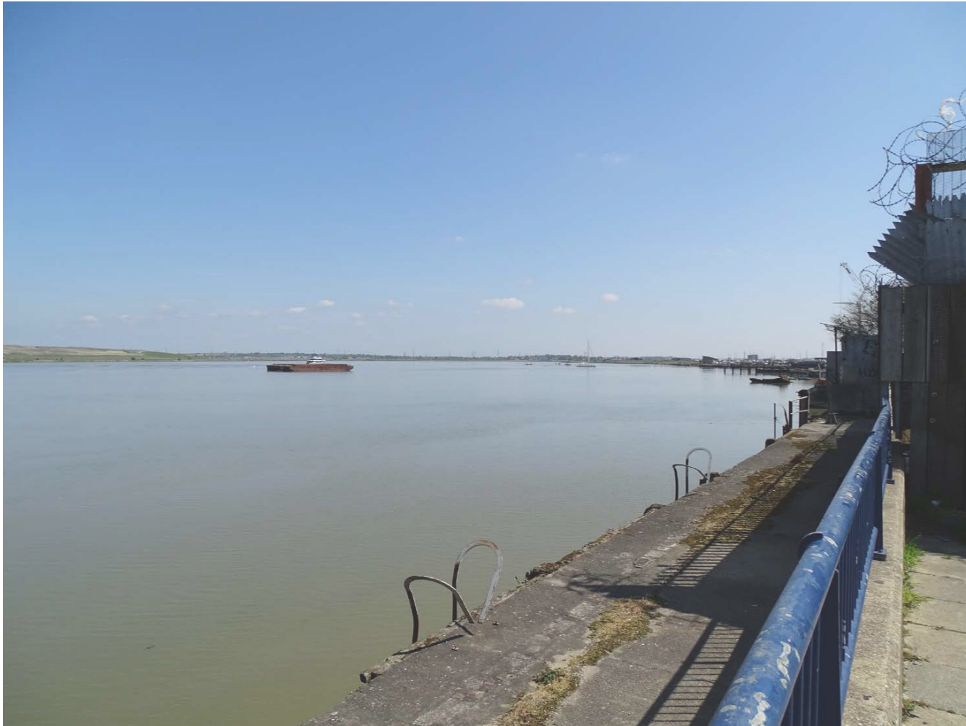
View East along the Thames - Path is blocked by an industrial estate.
