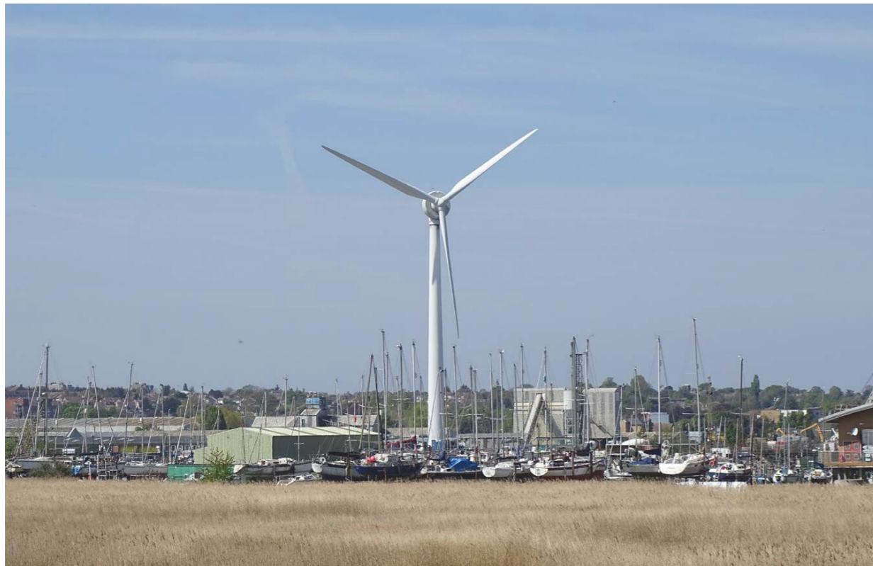
Wind Turbine in Erith.
