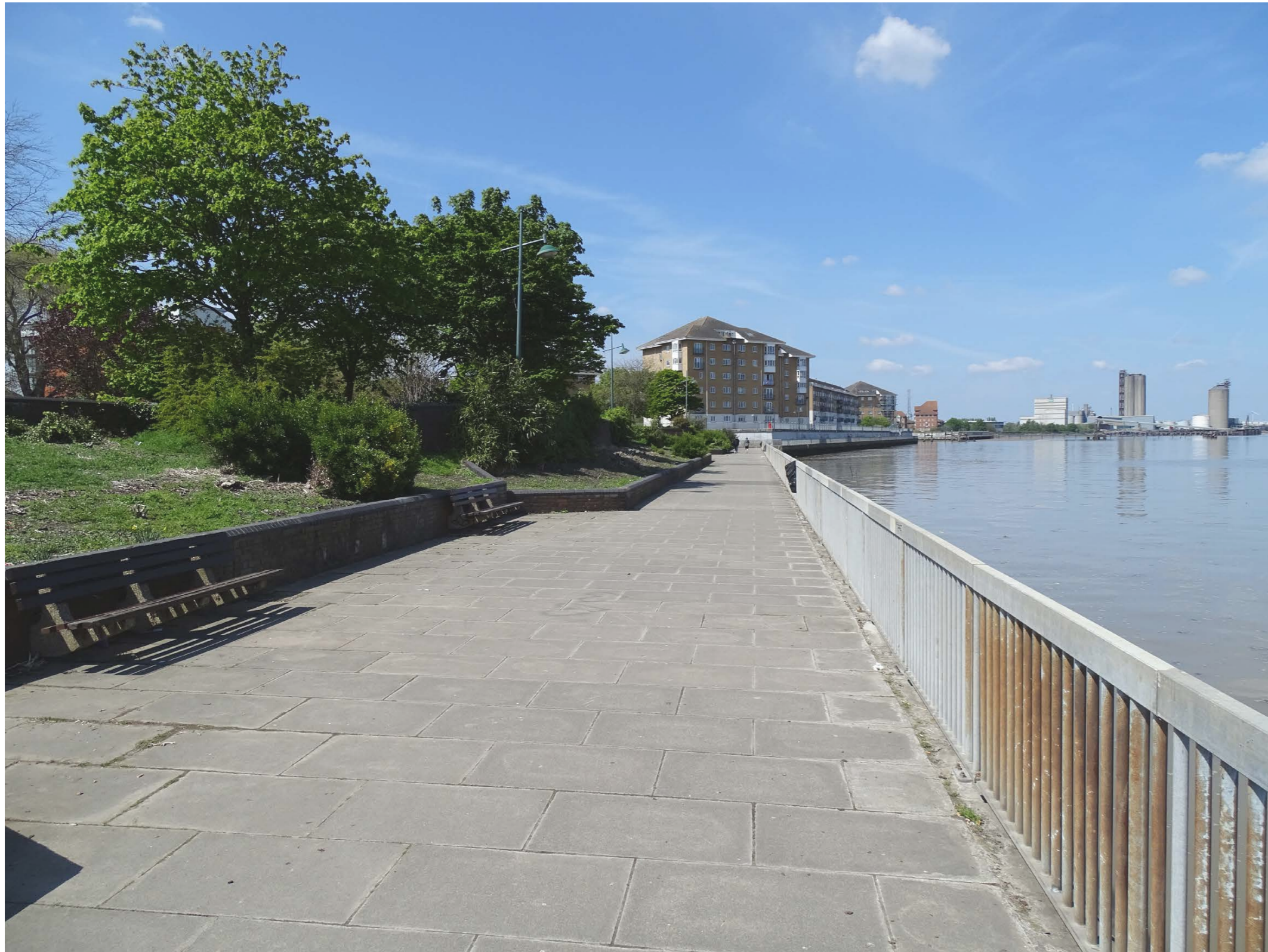
Existing Thames Path, Riverside Gardens, Erith - Improvements are to start soon.
