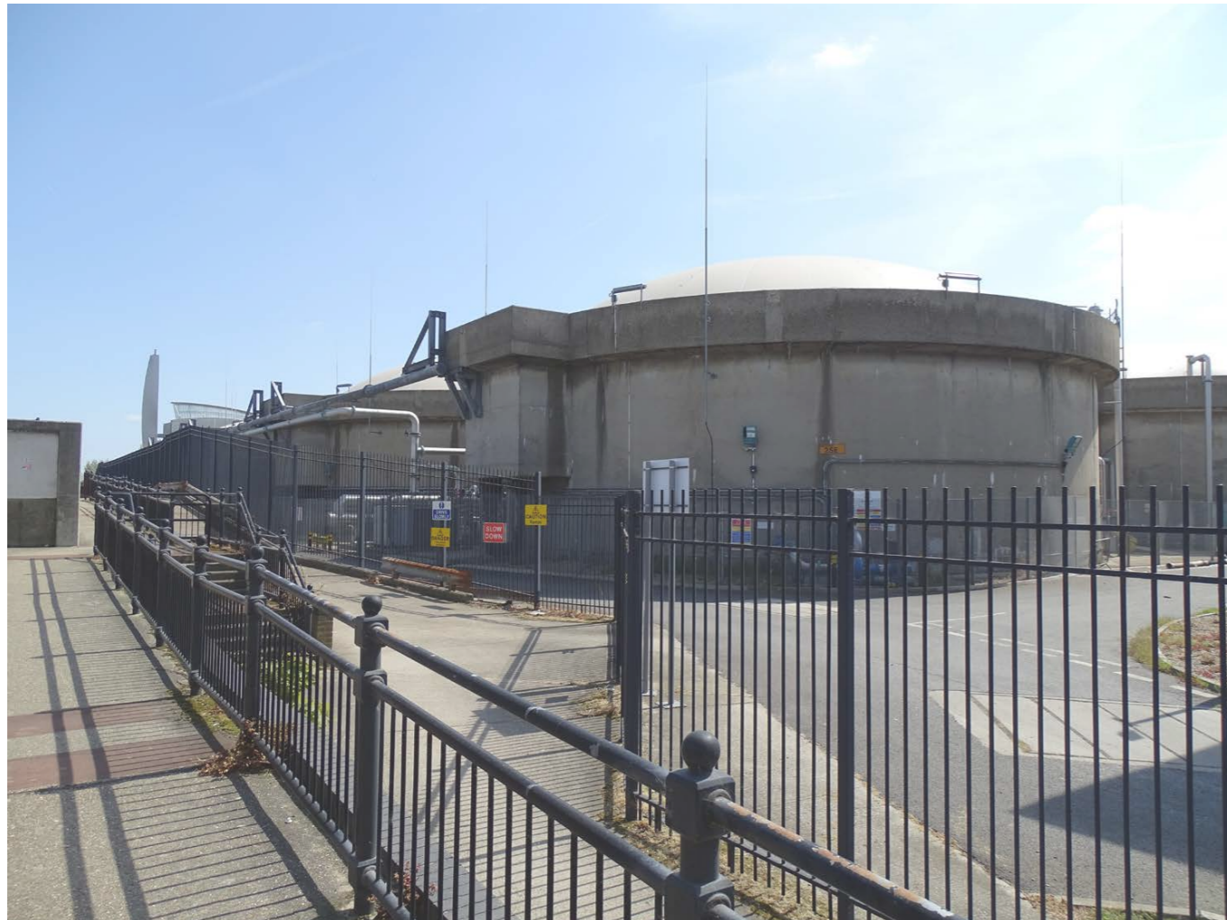
Crossness Sewage Plant
