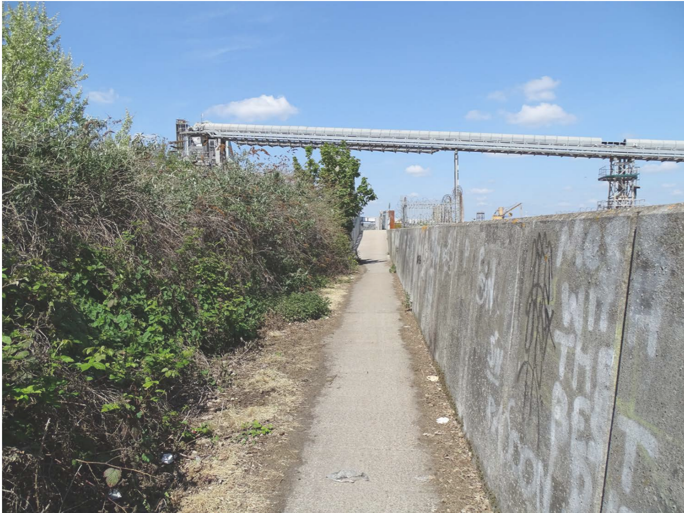
Thames Path alongside the Edible Oils process plant, Belvedere Industrial Estate.
