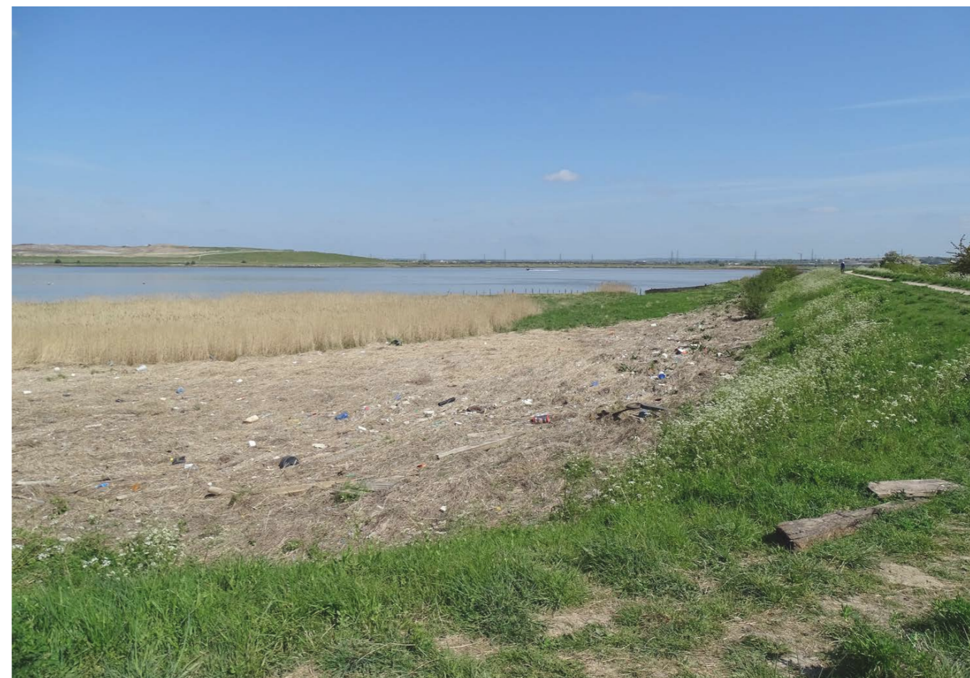
River bank next to Darent Industrial Estate, build-up of rubbish on river bank - View looking East.
