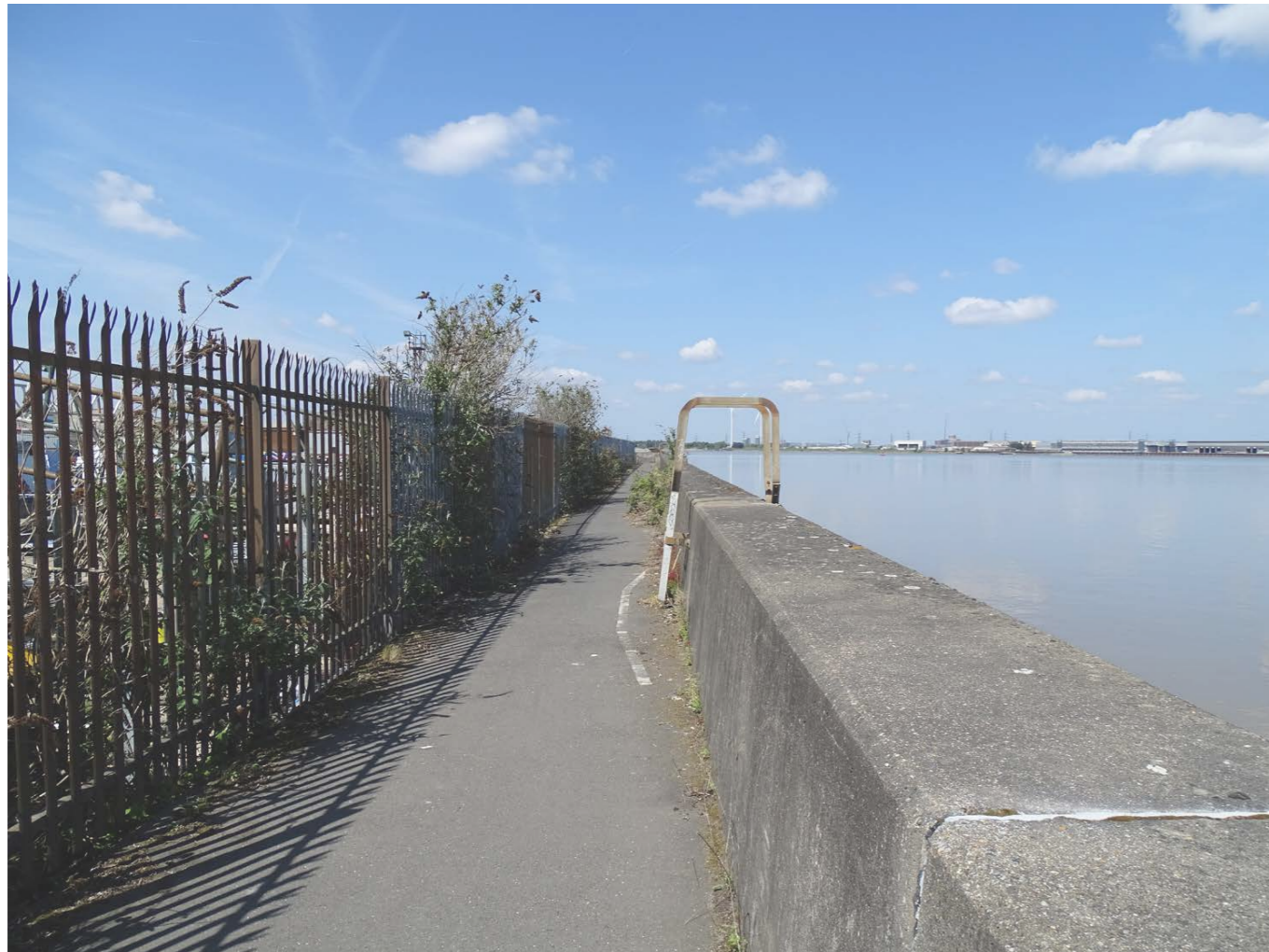
Metal railing fence at the boundary with Belvedere Industrial Estate.
