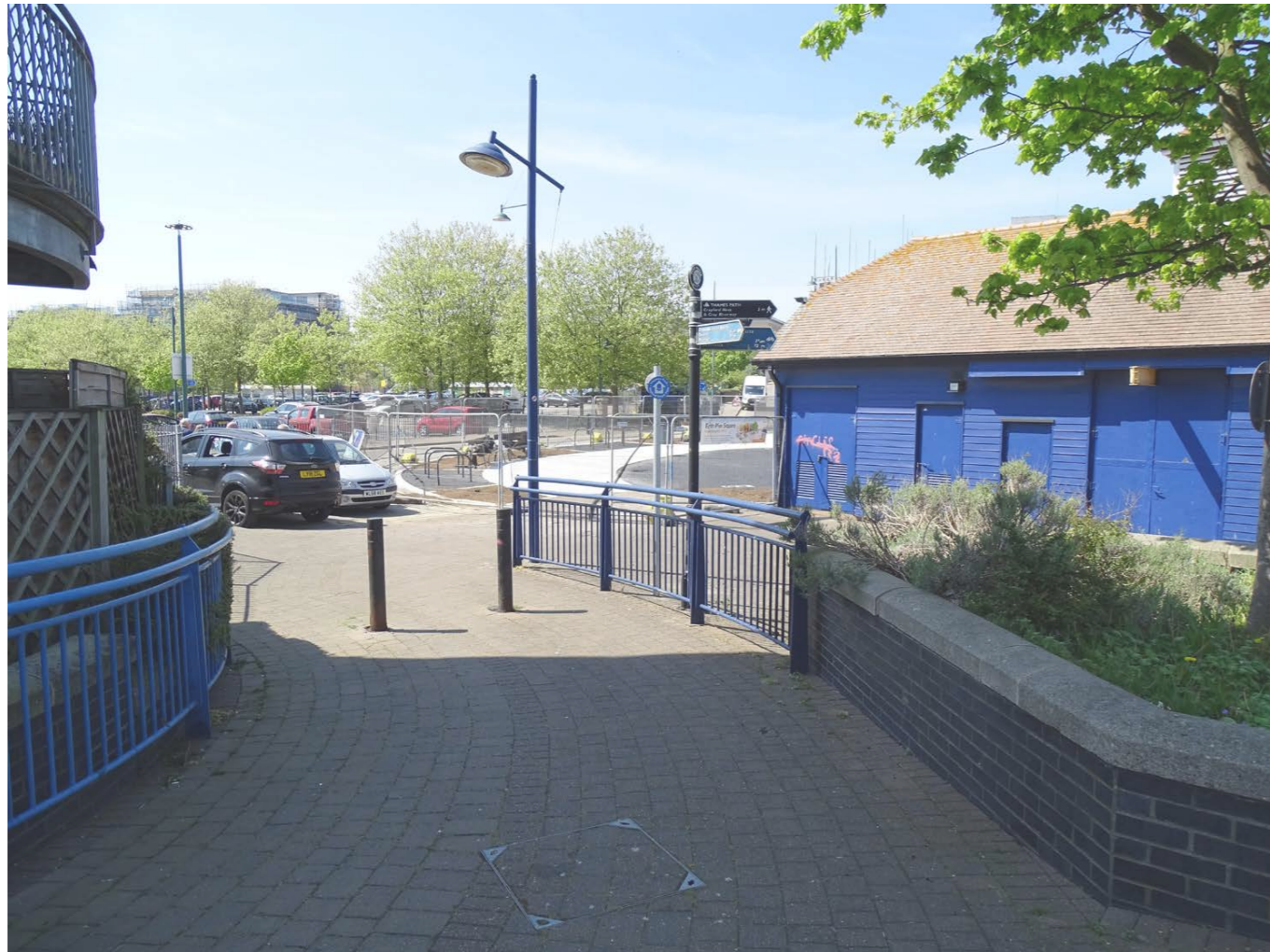
Base of Erith Pier - Currently undergoing improvements.
