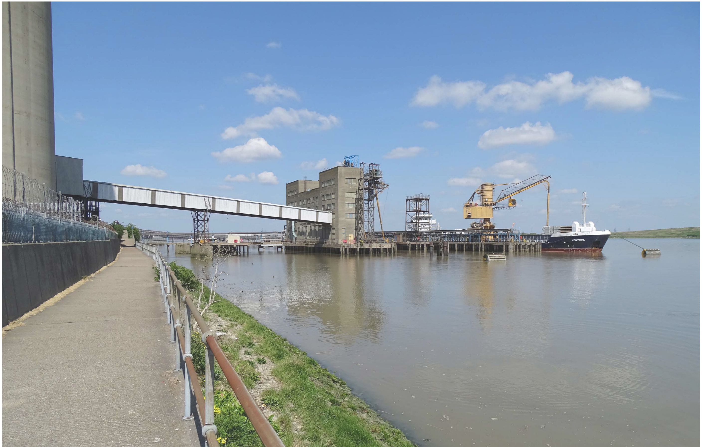
Oliver oil processing docking facilities - Belvedere Industrial Estate - Thames Path has been maintained amongst riverside industrial uses.
