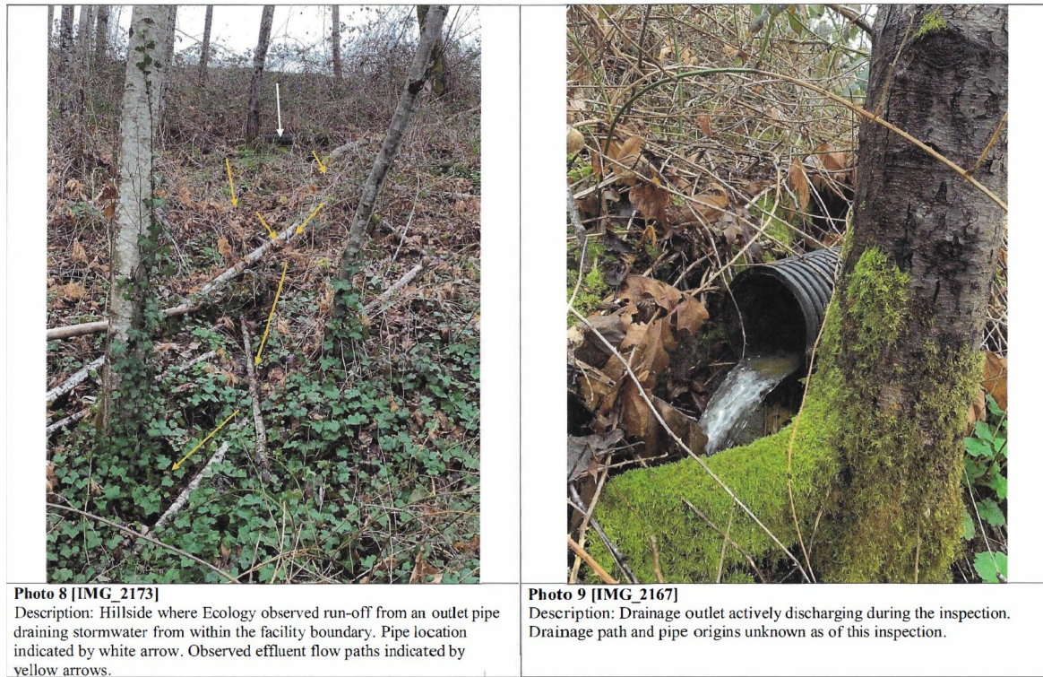
Figure 11: Photos 8 & 9 from Jay Fennell's, Dept. of Ecology March 21, 2022 inspection report. The pipe size was not noted but appears to be either a 12" or 18" N-12 HDPE pipe, flowing at an estimated 1-cubic foot per second.
