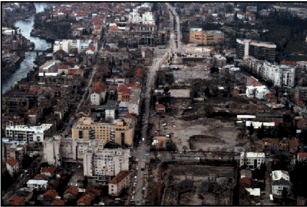
Figure 2-5. Close orderly block construction.
