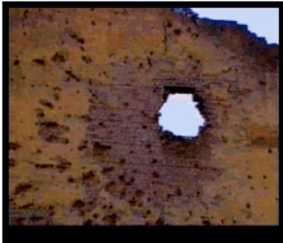
Figure 7-19. Examples of penetration and damage to buildings.
