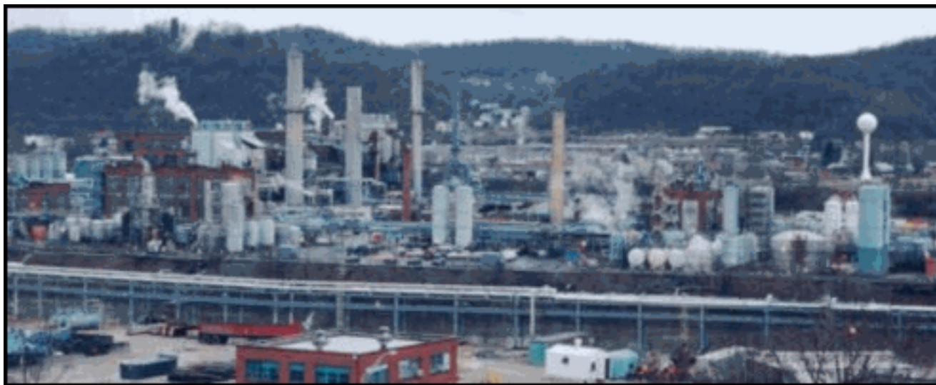
Figure F-1. Large urban chemical manufacturing plant.
