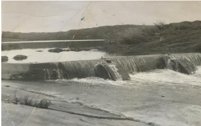
Picture of the spillway taken July 1960
