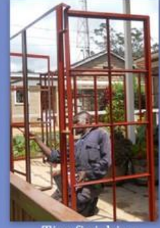
Tim finishing the windows
