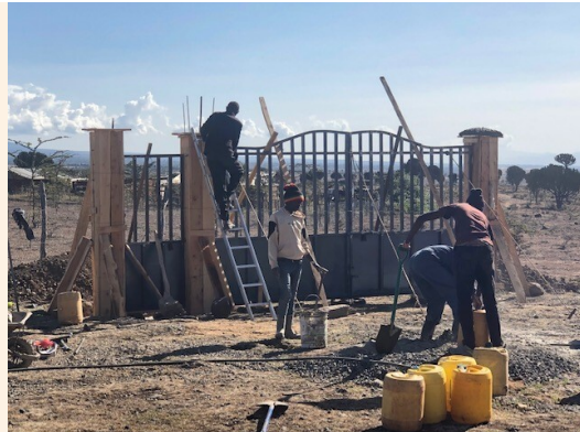
This month the JFM School gate was built and installed! The chain link fence was also finished!
