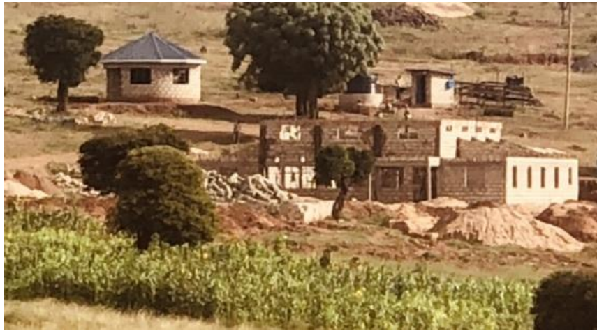
The JFM Angel Hill Mission Center/Headquarters is in the foreground. The mission bungalow, the water tank and pump house are behind the center.
