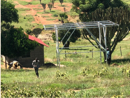
Solar tower and pump house
