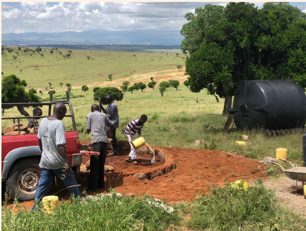
10,000-liter water tank
