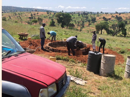
Water tank platform being built
