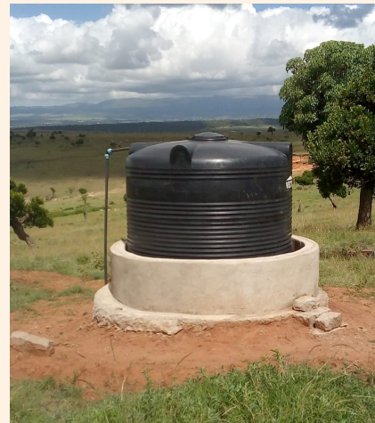
Water tank in place and pipes laid to well
