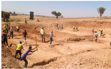
MISSION CENTER CONSTRUCTION IN FEBRUARY 2023
