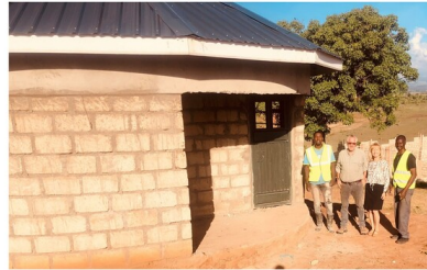
MISSION BUNGALOW CONSTRUCTION IN JUNE 2023
