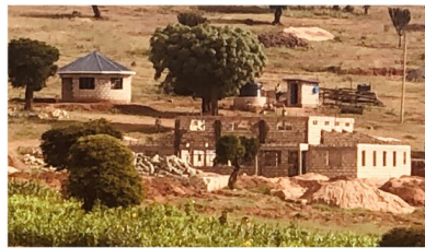
MISSION CENTER CONSTRUCTION IN JUNE 2023
