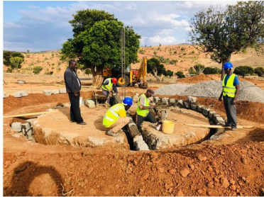
MISSION BUNGALOW CONSTRUCTION IN FEBRUARY 2023
