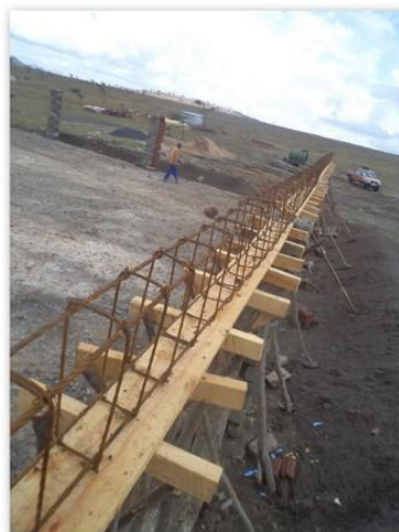
Lintel Framework Construction
