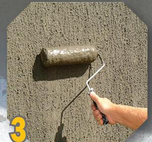
**3** Apply **BOND KOTE**, ensuring application is uniform in thickness and texture.
