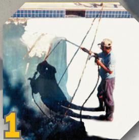
**1** Clean Substrate. Remove loose, delaminated plaster and contaminants.
