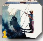
Clean Substrate. Remove loose, delaminated plaster and contaminants. Mix BOND KOTE properly.
