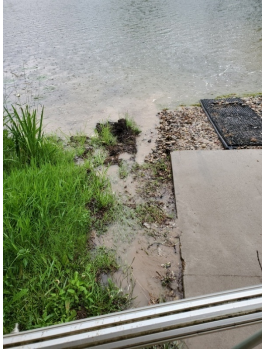
Minor erosion on northeast side of boat launch.
