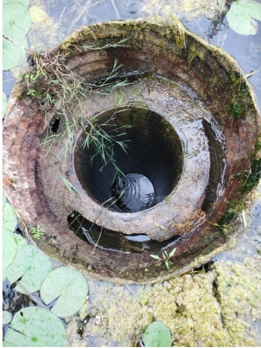
Looking down at principal spillway drop inlet.
