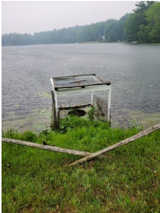
Principal spillway with a screened trash rack over the drop inlet.
