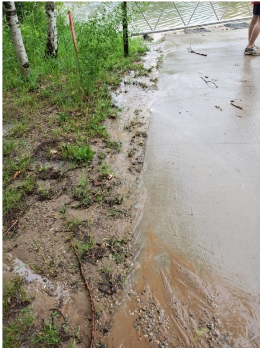
Channelized road runoff on northeast side of boat launch causing erosion.
