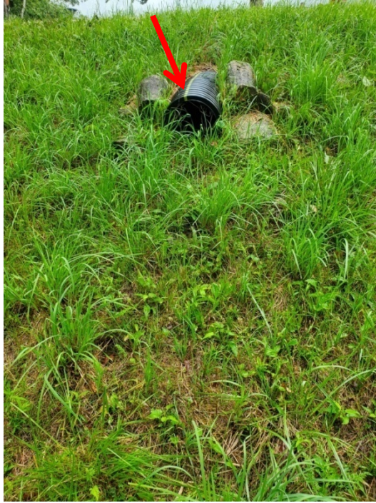
Downstream side of earthen embankment looking east shoing secondary spillway outlet.
