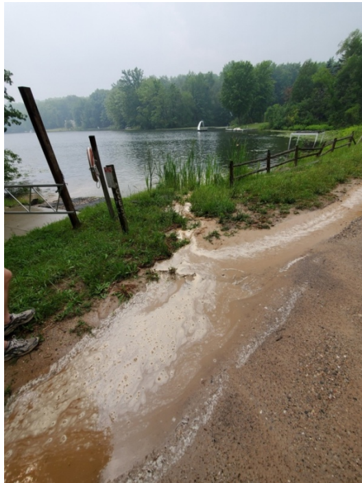
Channelized road runoff on southwest side of boat launch causing minor erosion.
