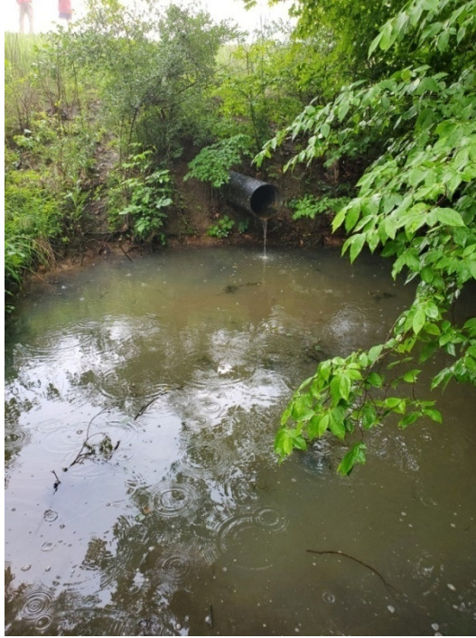
Plunge pool area at outlet of principal spillway
