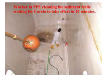
Incrustation begins to dissolve and surfaces sterilized as Carela is applied by spray
