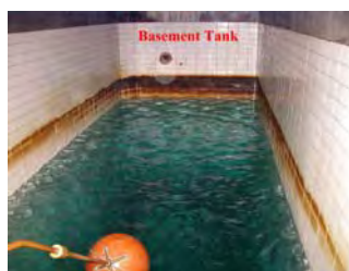
Incrustation deposited on the internal surfaces.
