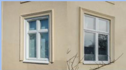
Before and after a window replacement - t.r. a new aluminium window t.l. the old wood window. Photo of a building in Nyköping, taken by David Hansson, Sörmlands museum.
