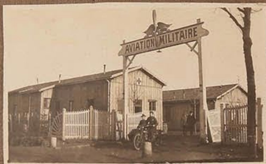
Tours Entrance to Camp May
