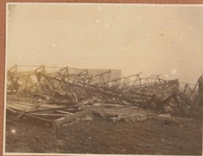
Wrecked Hangar Orly 1918
