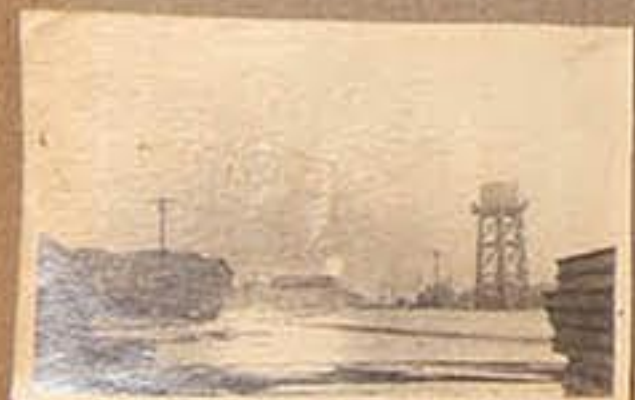
"The End of a Perfect Day" Digging Ditches - Shoveling Cinders - Flying Wheel barrows Issoudun Dec. 1917 25 Meter 1918
