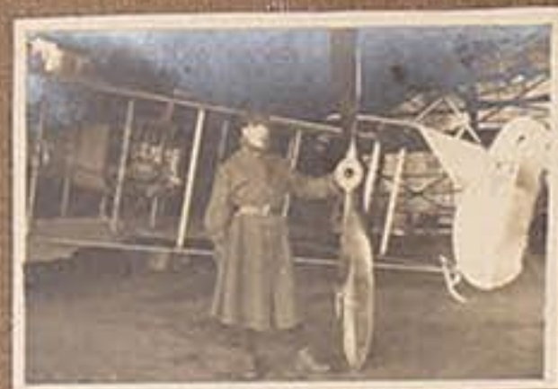
Farman 'Prop' Flew off 300 Meters Pilot and Machine Uninjured
