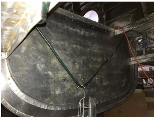
Wall to the lower turret
