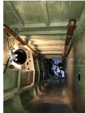
Hand Rails Installed
