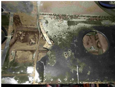
Wall on radio operator's floor prior to repair
