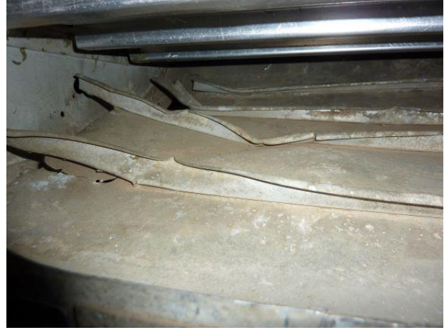
Buckled skin seen from inside plane
