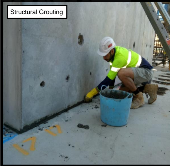
Concrete Repairs
