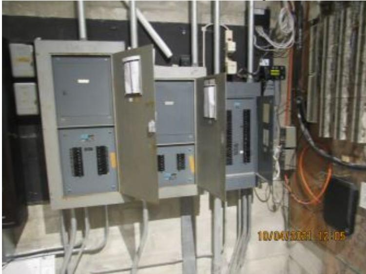
**Photo 5: Main electrical room. Electrical panels (Zinsco)**
