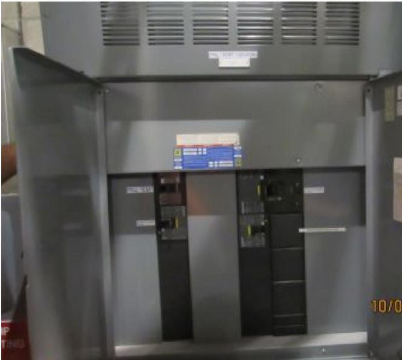
**Photo 4: Main electrical room-Emergency distribution panel**
