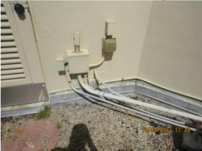
**Photo 24: Roof-Exposed cables**
