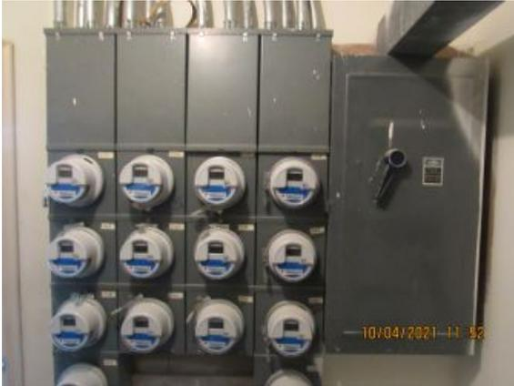
**Photo 17: 600A Zinsco Meterbank with 600A disconnect (Typ meter room,3<sup>RD</sup> floor, 5th floor,7th floor, 9<sup>th</sup> floor, Penthouse)**
