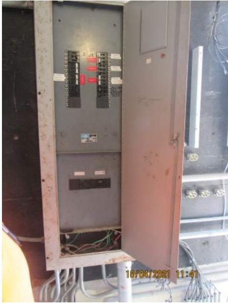
**Photo 22: Roof-Electrical room-Electrical distribution panel (Zinsco)**
