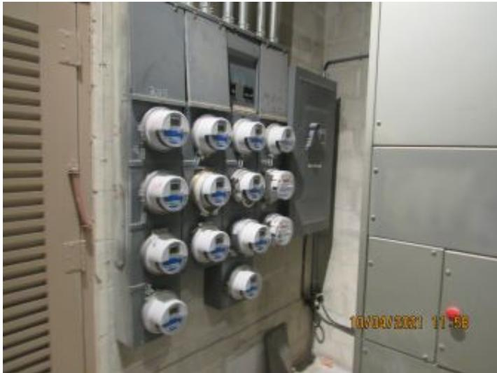
**Photo 2: Main electrical room- 600A Zinsco Meterbank with 600A disconnect**
