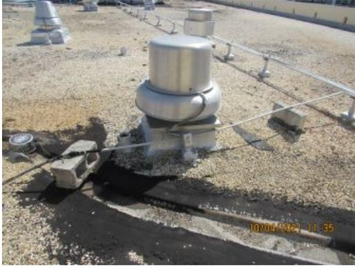
**Photo 19: Photo 18: Roof-Weatherproof flex conduit (Typ)**
