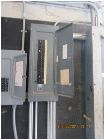
**Photo 23: Roof-Electrical room-Electrical distribution panel (Zinsco)**
