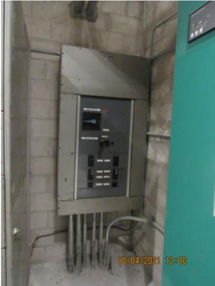
**Photo 3: Main electrical room- Electrical distribution panel (Zinsco)**
