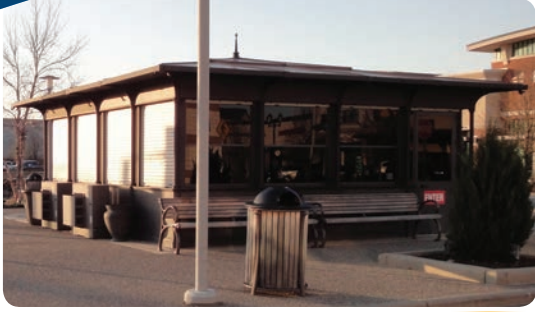
Enclosed Shelter House/ Public Restroom
