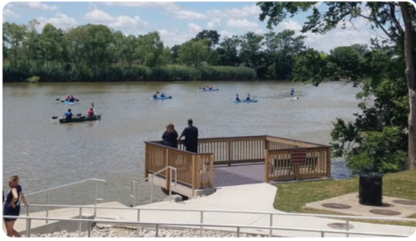
Seasonal Public Docks and Kayak/Canoe Launch Lookout Deck and Fire Dock -Completed Project
