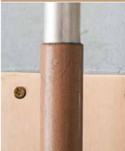
Close-up of the pull (after two years of use on the men's room door) prior to the most recent cleaning with Edelman Leather Cleaner.
